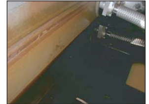
Typical operating gas turbine reservoir
