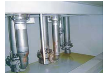
ISOPur BCA treated gas turbine reservoir after just 3 months
